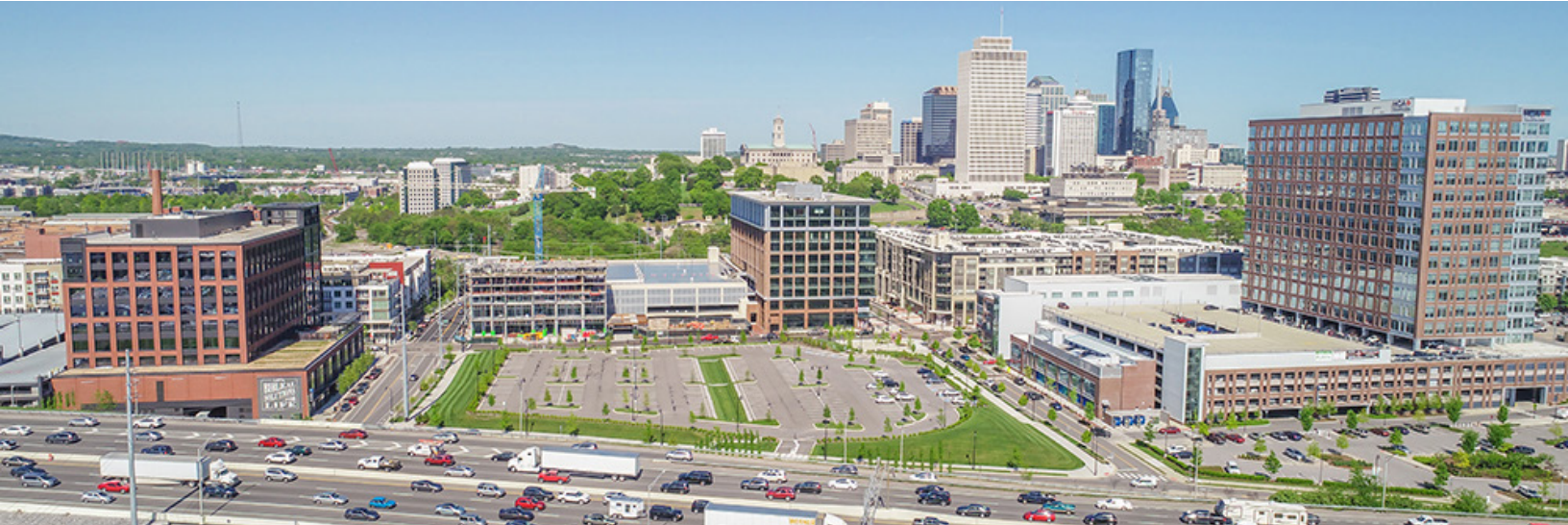
VIEW FROM 4TH FLOOR OFFICE TERRACE
