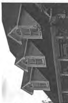
Don't: Typical tract house pork chop eaves project equally too far to the gable end as they do to the eave sides. Pork chop dormer eaves do exactly the same thing, accentuating the top-heavy appearance of the dormers.
