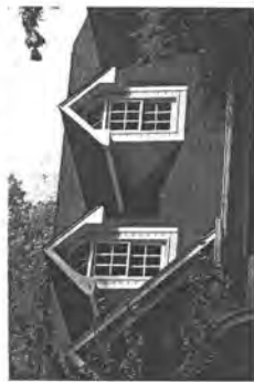
Don't: Circle-head windows jammed between pork chop eaves still leave blank slivers to fill with siding.
