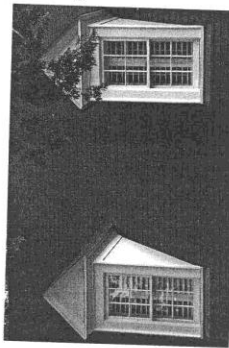
Do: The dormers on this fairly classical midrange building also have siding in the tympanum. Because refined than the first, the designer has used flush tongue and groove siding to make the joints less apparent.
