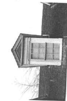
Do: This classical dormer has a small tympanum that is fitted with a single board, creating no seams at all.
