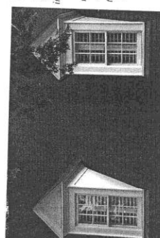
Do: The dormers on this fairly classical midrange building also have siding in the tympanum. Because this building is more refined than the first, the designer has used flush tongue and groove siding to make the joints less apparent.
